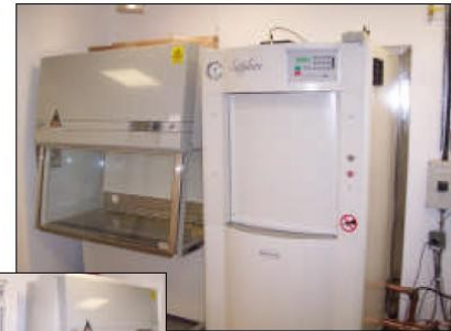
Shown here are both sides of a double ended autoclave installation.
